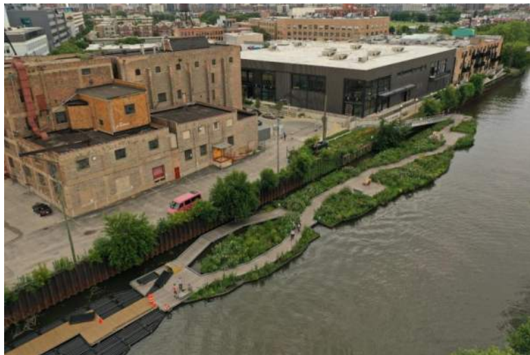
Constructed wetlands at River Point Park, Spokane (top). Floating wetlands in Chicago's Wild Mile .
