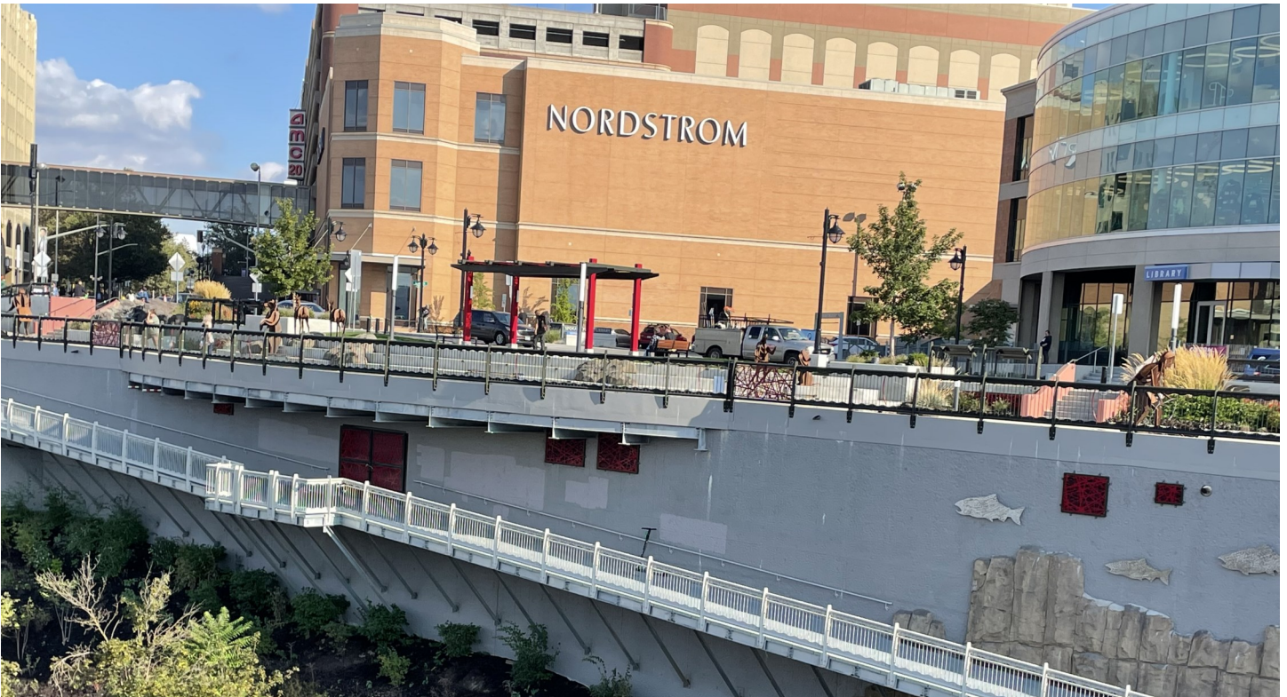
Combined Sewer Overflow Tank Spokane Falls Blvd.
