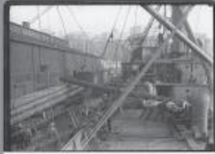
Image of Forklifts/Handcarts/Manual Lanes
