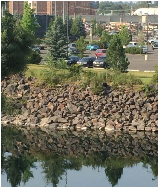
Rock Armor Slope at River North shore
